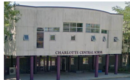
Charlotte VT Public School PH Certified Ventilation System Charlotte VT
